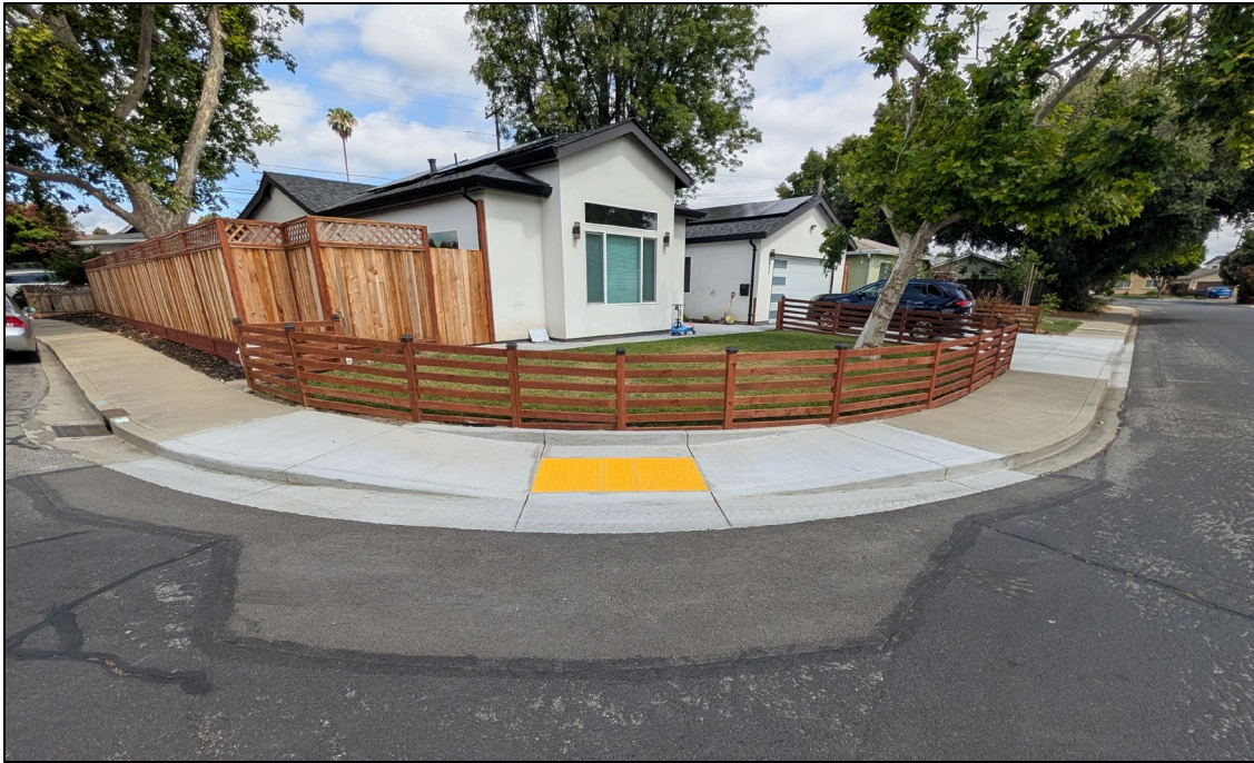
Curb Ramp Improvement
