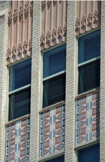
Color reinforces the role of the panels as decorative rather than strong and load-bearing.
