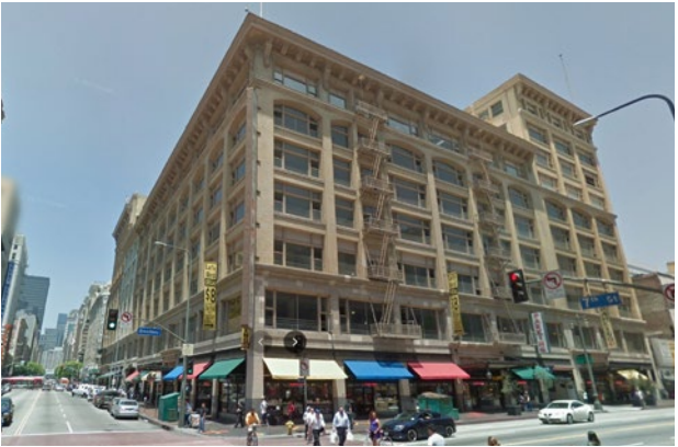
FLEXIBLE BUILDINGS like this example in downtown Los Angeles, whose upper floors once hosted a department store and offices but now serves as a parking garage.
