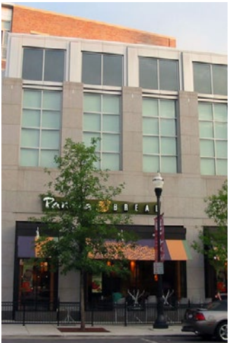
STACKING MATERIALS —Masonry used below lighter materials such as stucco, synthetic cladding, or siding.
