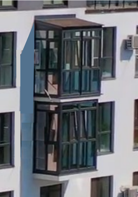
This modern bay window has a metal structural frame supported by concrete cantilevers.
